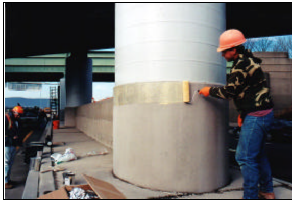
Roller Application of Adhesive
