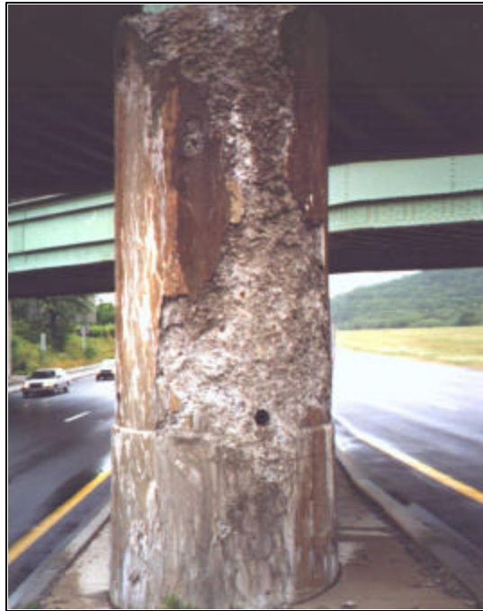
Bridge No. 7012680 and 7012690
