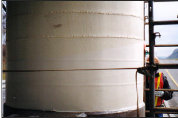
Spiral Wrapping in Progress
