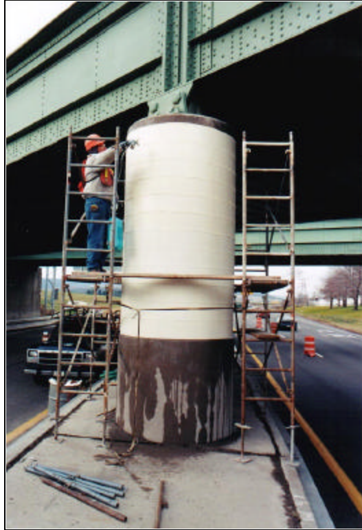
Completing the Structural Layers
