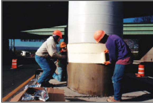
Structural Layer over Adhesive
