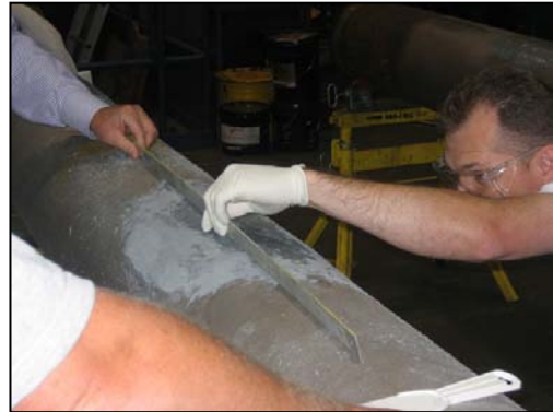
Fig. 4 – Use a straight edge to confirm evenness.
